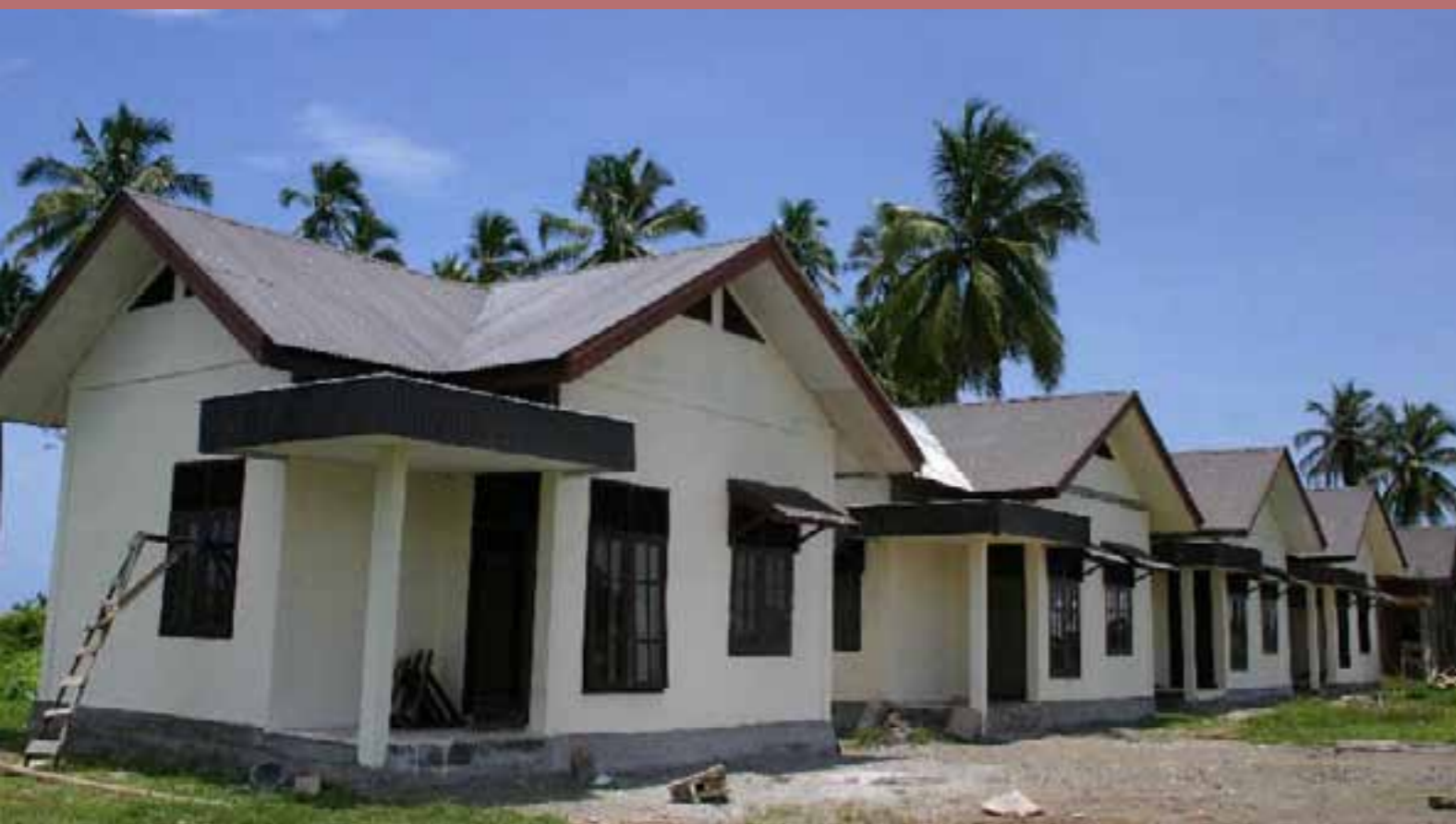
Islamic Relief has constructed 194 earthquake-resistant houses in Suak Pandan village for those made homeless by the tsunami
